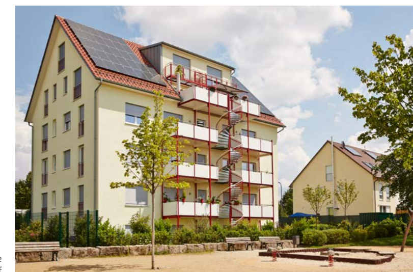
Exterior view of a new low-energy house with a photovoltaic system on the roof
